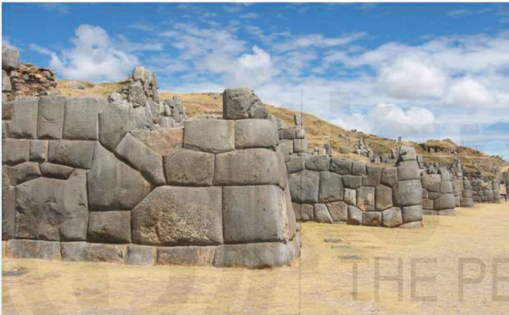
Figure 11.5: Walls of the Sacsayhuaman Ruin at Cusco (Ashlar Polygonal Masonry)
