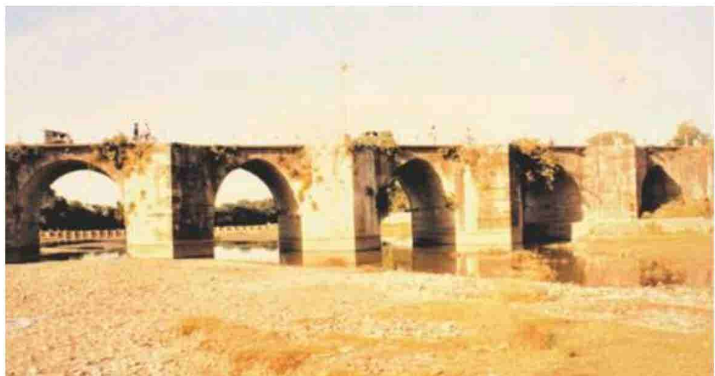
Figure 18.17: Bridge Over Gambhiri, Chittorgarh Photograph: Ravindra Kumar
